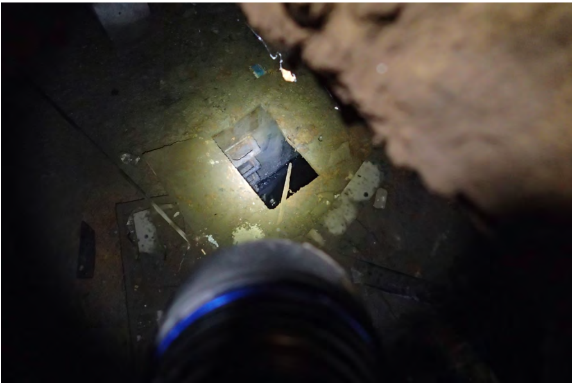
Photo 18: Stoking floor sump access. Photo taken through floor penetration.
