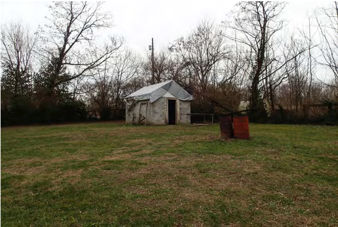
Photo 26: Storage building at law enforcement shooting range.
