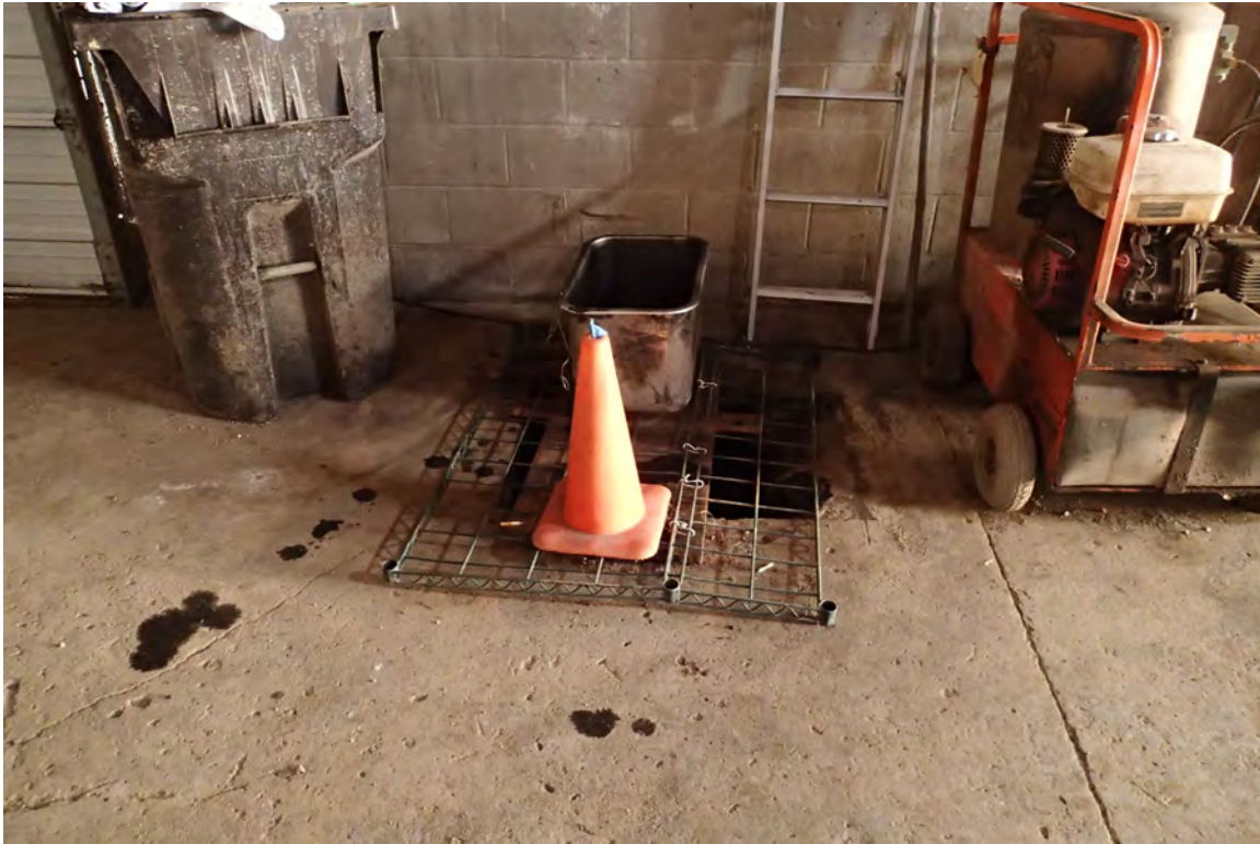
Photo 13: Entry location to confined space area under building floor.
