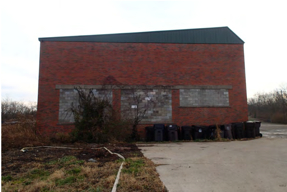
Photo 4: View of west facing side of building.
