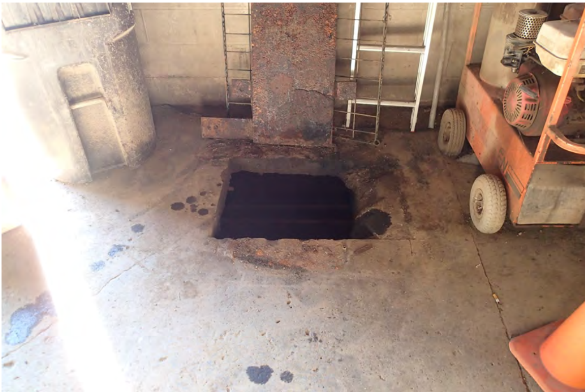
Photo 14: Entry location to confined space area under building floor.
