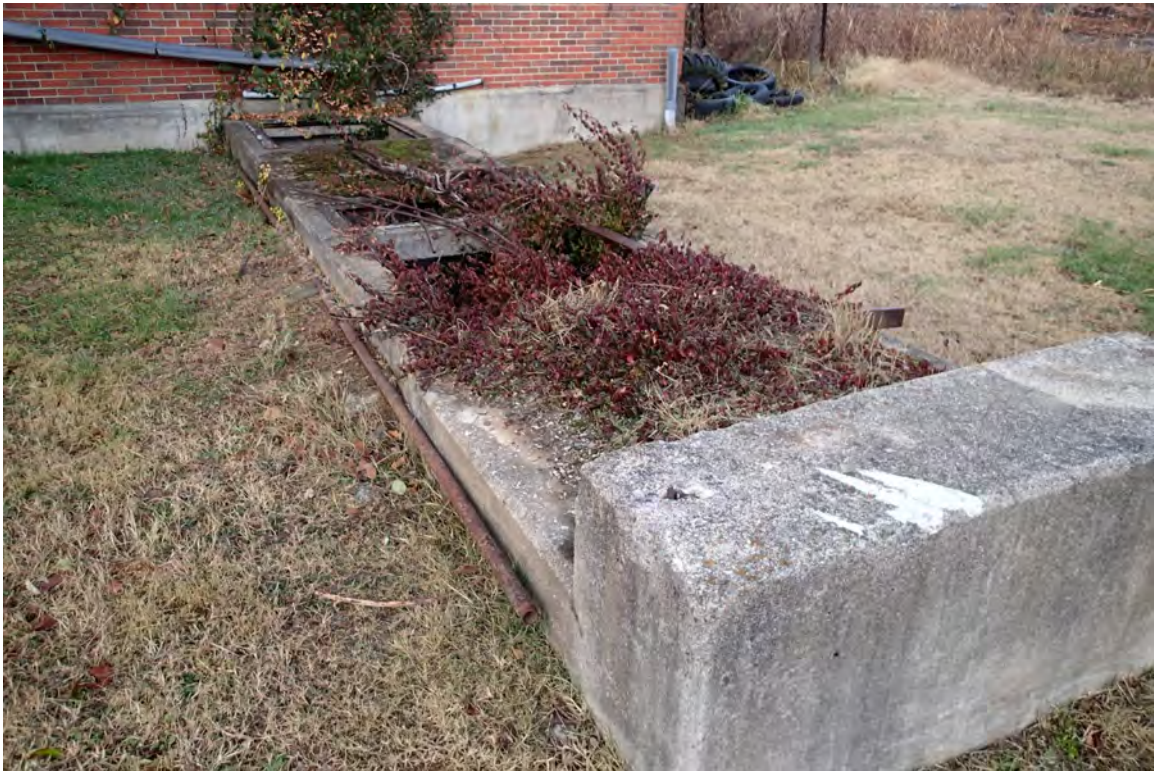
Photo 7: Remnants of ash removal conveyor, east incinerator.
