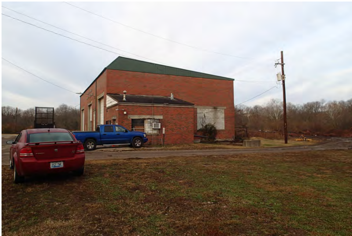
Photo 2: View of the east facing side of the building.
