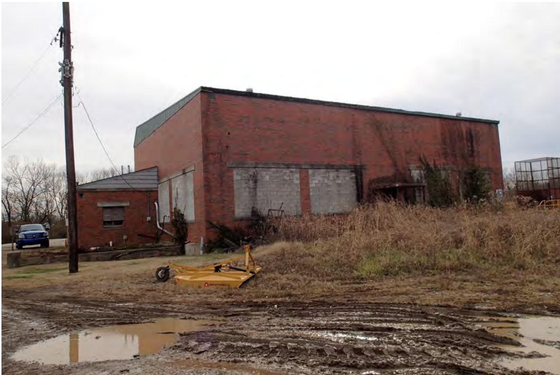
Photo 3: View of north facing side of building.
