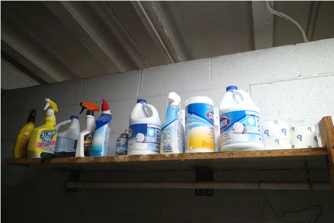
Photo 19: Cleaning chemicals stored in bathroom.
